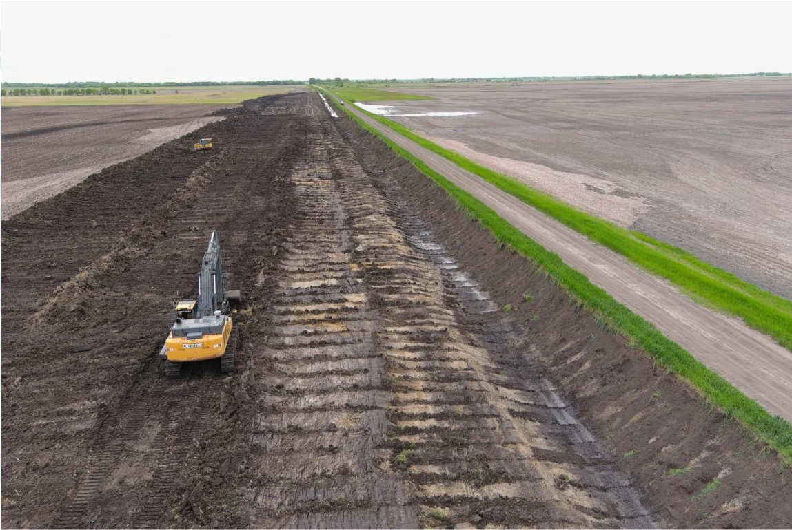
06/07/22: Topsoil Stripping
